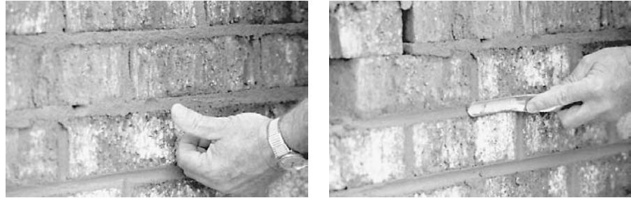
Figure 15-23 Concave tooling when the mortar is “thumbprint hard” should produce joints of uniform color and appearance that are well compacted at the bond line to maximize resistance to water penetration. (Photos courtesy BIA.)
